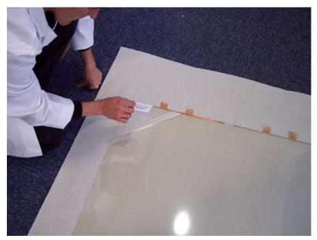
Using the edge tab of the label remove the first 100mm (4") of the protective liner covering the cling side on the bus-bar edge. Make sure that you do this in a clean dust free environment.
