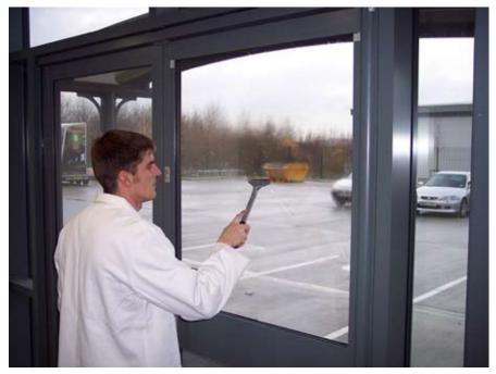
Spray the glass with liquid glass polish and use a window scraper or blade to remove any dirt / blemishes from the glass surface.
