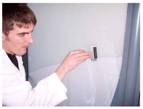
Gradually pull away the protective liner and allow the film to slowly adhere to the glass surface under its own pressure. Using the roller move down the film working in horizontal lines left to right to disperse any air bubbles. If any small bubbles are visible, carefully lift the film and let it sit back down under its own pressure.
