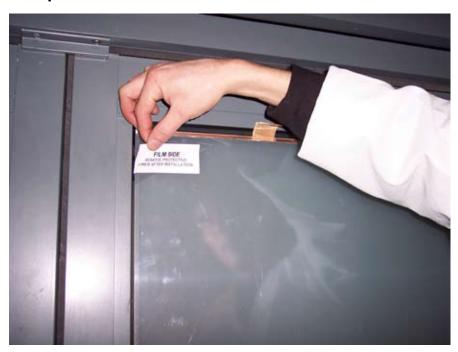
You can now lift the tag and carefully remove the protective liner.
