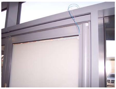
Run some clear double sided tape along the bus-bar edge to hold your electrical cables in place while you prepare the cover trim.
