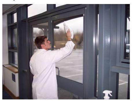
Spray the glass with liquid glass polish and clean with a soft lint-free cloth. Repeat this process until you are sure that the surface is completely clean.
