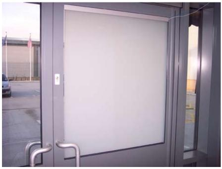
Your installation is now complete and you can clean the film using either liquid glass polish or IPA cleaner and a soft lint-free cloth. For most installations we would recommend that you use a cover trim on all edges of the film.
