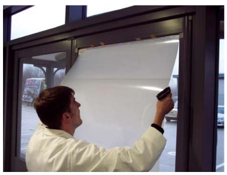
Align the bus-bar edge of the self adhesive Intelligent Film with the top edge of the glass. When in position run your finger along the bus-bar to fix the top edge (the adhesive strip will hold the film in position).
