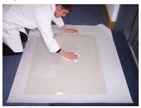
Wipe down the protective liner on the cling side of the self adhesive Intelligent Film to remove any dust.
