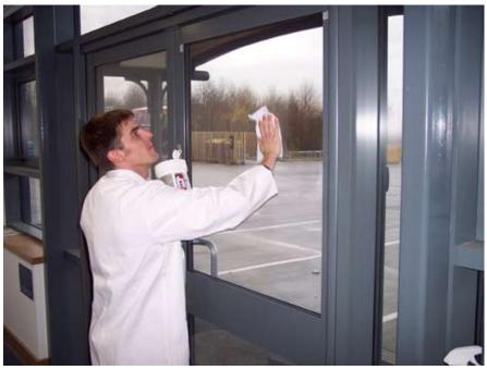
Using a lint free cloth, wipe the glass surface with IPA (Isopropyl Alcohol) and leave to evaporate.
